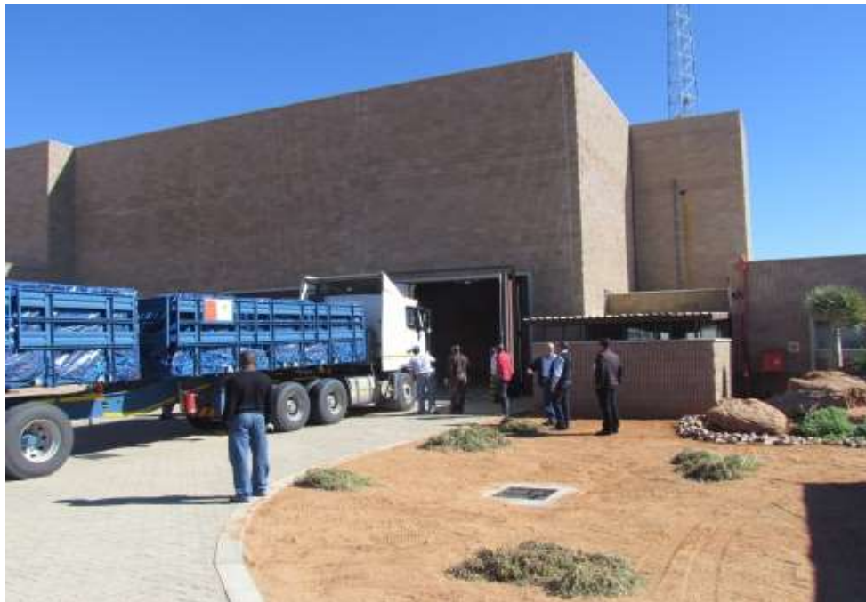
Figure 4: Arrival of Waste at Vaalputs
