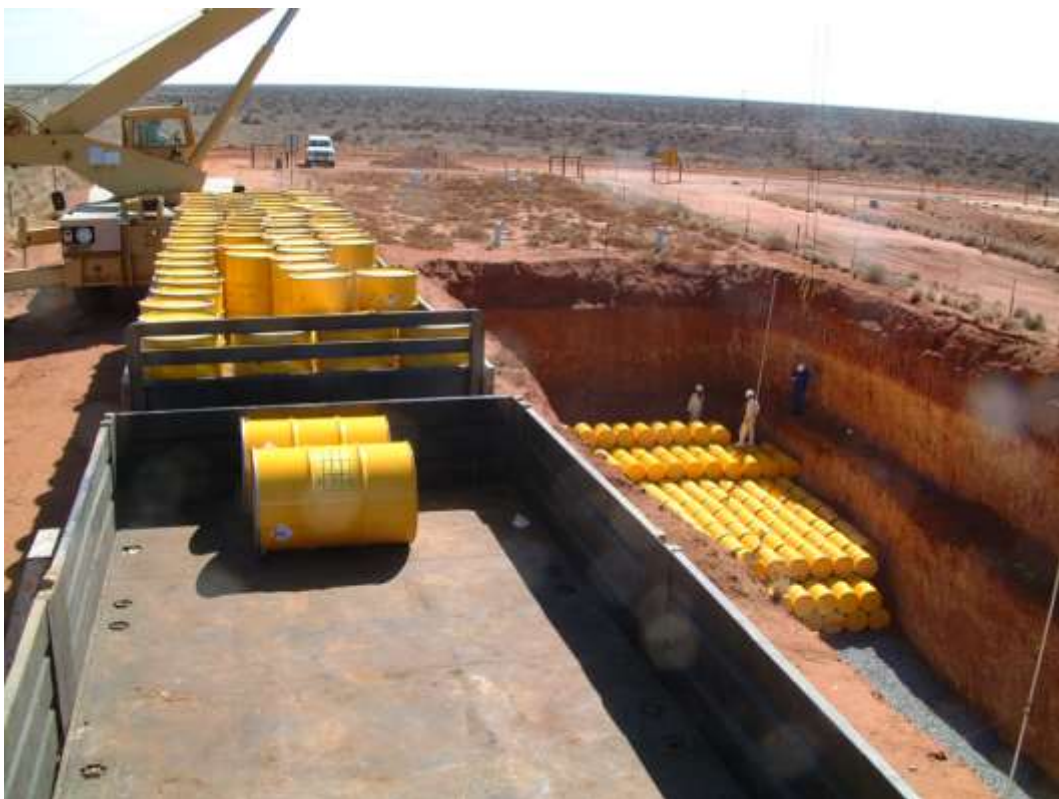
Figure 3: LLW metal containers being emplaced in a disposal trench
