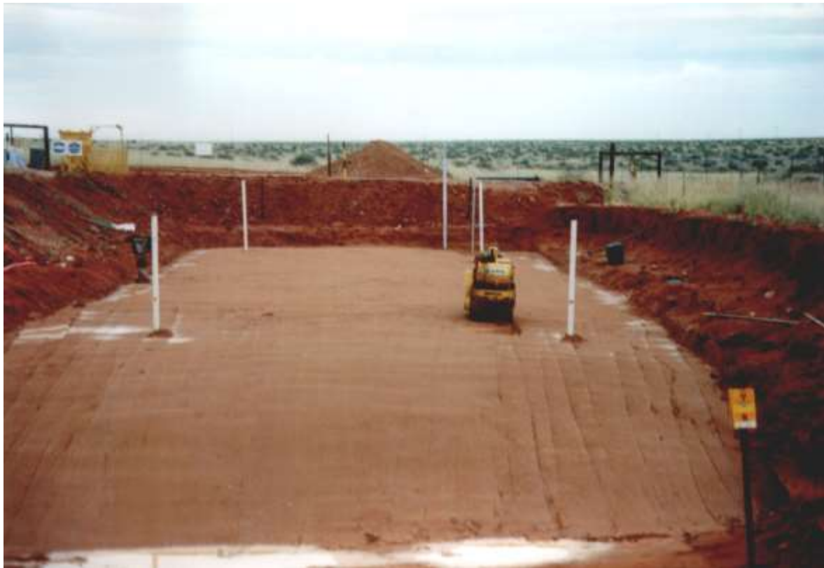
Figure 8: Capping of Disposal Trench
