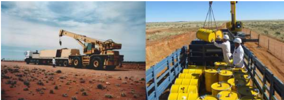
Figure 6: Disposal into trench
