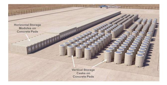
This storage system uses a dual-purpose canister (DPC) where SNF assemblies are placed into a welded sealed metal container which provides the primary confinement boundary for the SNF. The DPC is placed in different overpacks or casks, which provide radiation shielding and physical protection, during canister transportation, transfer, or storage. A typical PWR canister will hold 24 to 37 PWR SNF assemblies.
